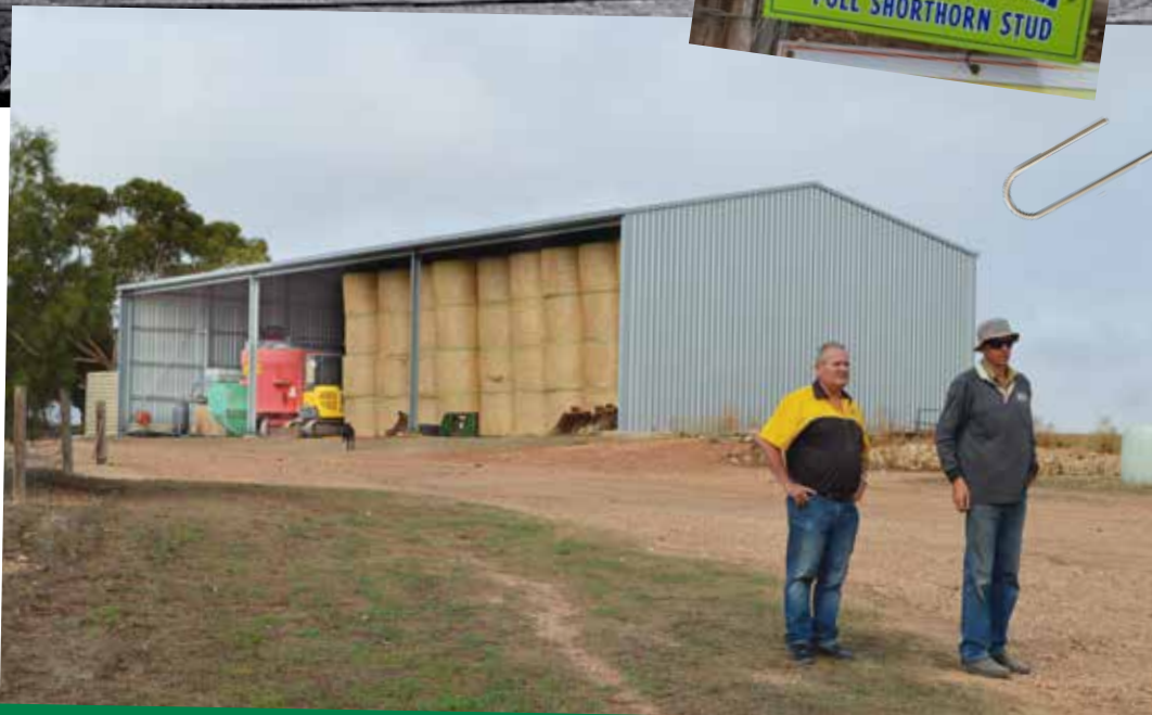
Grant Sheds owner Danny Halupka checks out the coastal views with Ardrossan mixed crop and livestock farmer Ashley Rowe. The hay shed behind them has 3 x 9m wide bays for easy access.
