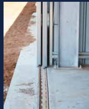
They chose bottom roll sliding doors - very easy to roll open despite large 6m x 5.1m size..
