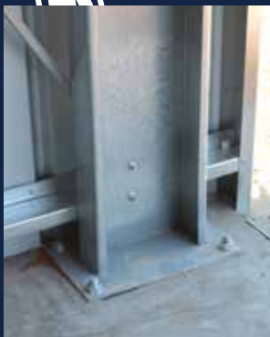
Strong connection to ground via heavy baseplates & large footings bolts.
