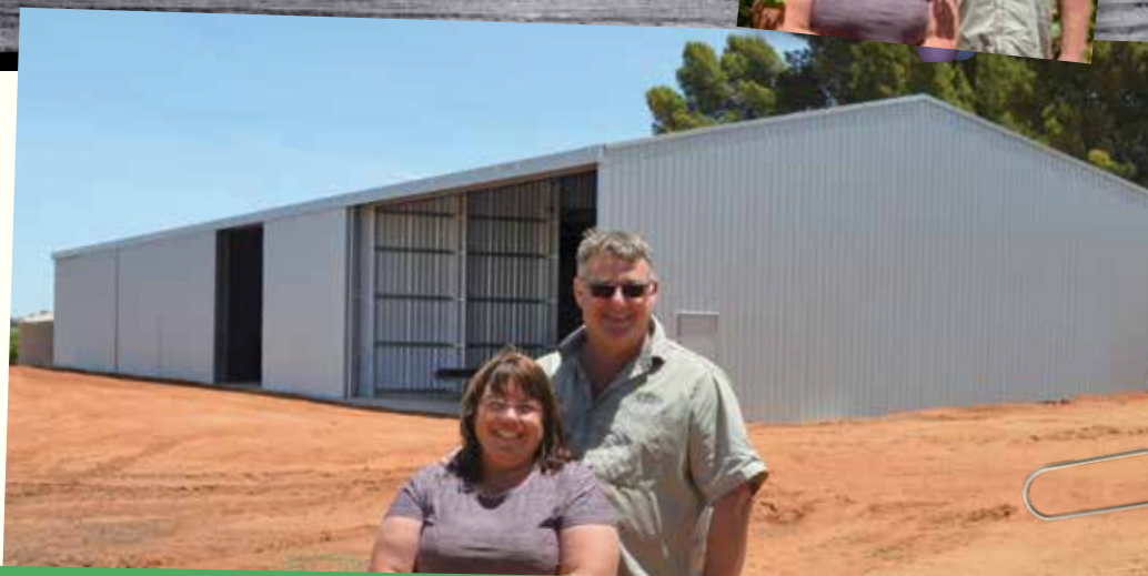
Jacque & Peter Schulz are proud of their new Grant Sheds machinery shed. It's 15m x 48m x 5.1m with 4x12m wide beams so they have minimal front columns, 8/6m wide x 5.1m high bottom roll sliding doors and a partition wall inside the shed to create a workshop area.
