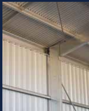
Strong Super-C frames and solid X-bracing creates a well braced, solid shed.
