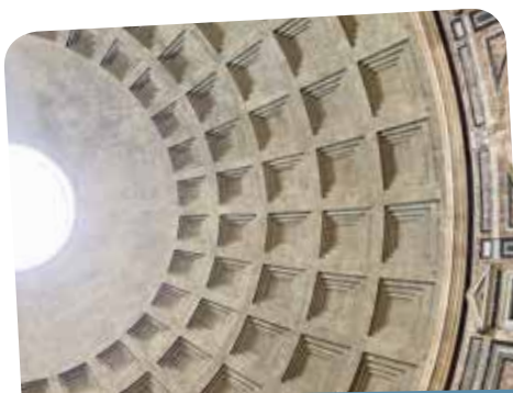
Looking up at the coffered concrete dome roof and central roof opening in the almost 2000 year old Pantheon building in Rome.
