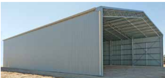
20m x 30m x 6.6m MEGA Shed
