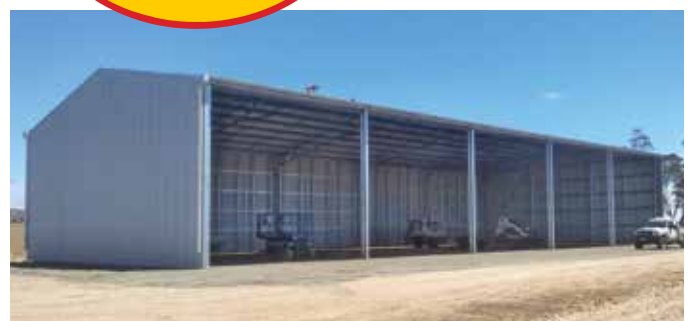
18m x 40.5m x 7m MEGA Hay Shed
