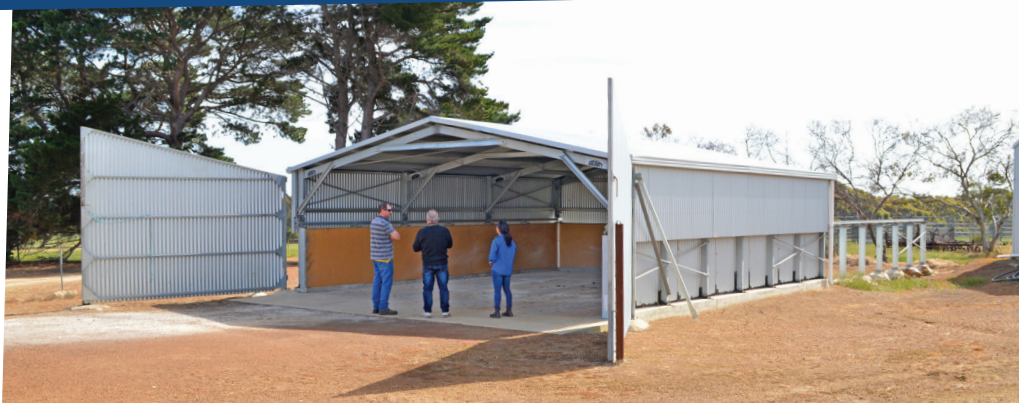
Ready to fill! Danny with Damien & Annette in the Sliding Roof Bulk Fertiliser Shed. The optional swing doors are open here. Two people can easily push the roof back onto the runout tracks behind the shed. It only takes 5-10 minutes to unload a semi-tipper truck, including opening and closing the roof! In fact, we timed it, it took just one minute to open the roof (photo below shows open position) and another one minute to close it. Then there's just the truck reversing and tipping time.
