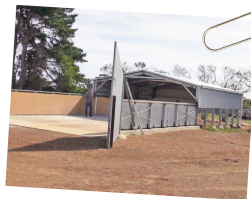
Ready to fill! Danny with Damien & Annette in the Sliding Roof Bulk Fertiliser Shed. The optional swing doors are open here. Two people can easily push the roof back onto the runout tracks behind the shed. It only takes 5-10 minutes to unload a semi-tipper truck, including opening and closing the roof! In fact, we timed it, it took just one minute to open the roof (photo below shows open position) and another one minute to close it. Then there's just the truck reversing and tipping time.
