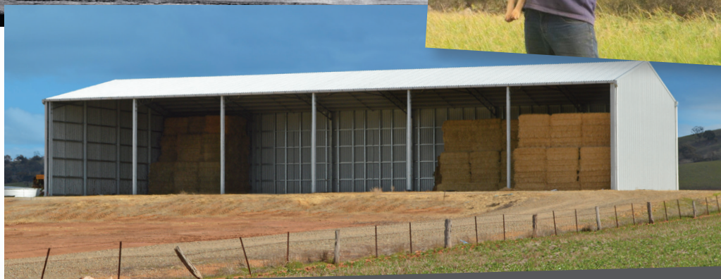
The Stephenson's 24m x 48.6m x 8.2m Grant Sheds MEGA Hay Shed holds 3250 high density large square bales of hay. It fits 9 bales high (& 10 high at the centre of the gable) which suits 3 lifts of 3 bales per lift with their manitou. The 8.1m wide bays is ideal for 3 bales per bay.
