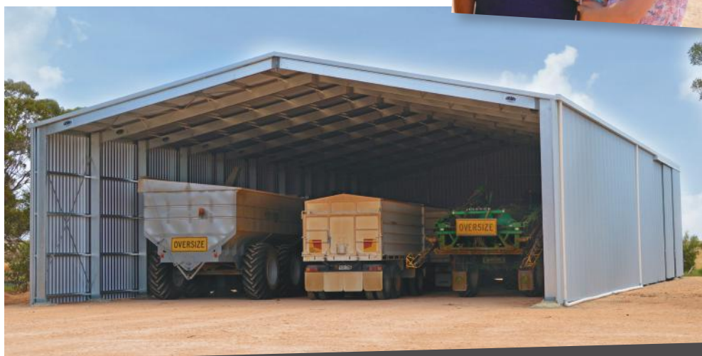
The newest "Grant" shed in the Niejalke family collection is this 15m x 30m x 5.1m Machinery Shed to protect their valuable farm vehicles and machinery.
