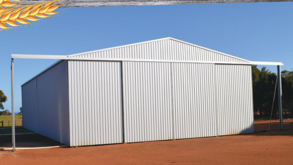
Peter Wake's new Grant Sheds machinery shed was purpose-designed to accommodate his farm's large machinery and gives an easy, drive-through and cost-effective solution. Easy-roll sliding doors & outriggers on this end allow full width opening of the shed and protection from prevailing weather direction.
